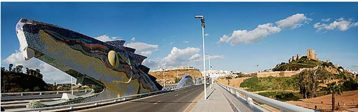
The bridge itself is made up by two roads of 7 metres each one with two lanes 3.5 metres wide each, two 2.5 metres sidewalks and a central 3-metre wide central reservation. The structure emulates a dragon that gets out of the Castle hill crossing the River Guadaíra, at the foot of one of the largest Almohad fortresses in Europe. This way, the dragon is "the Guardian of the Castle" and the town defender, and also the one in charge to receive its visitors.
